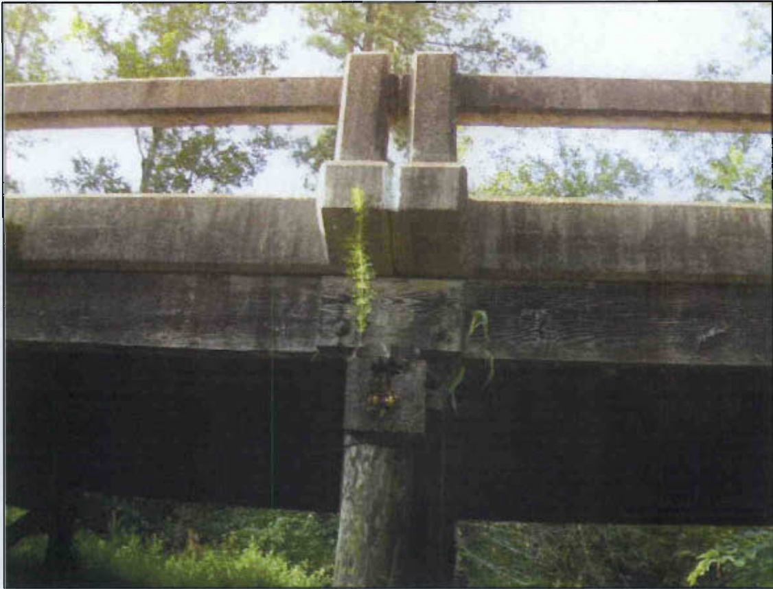
NORTH END OF BENT 1
