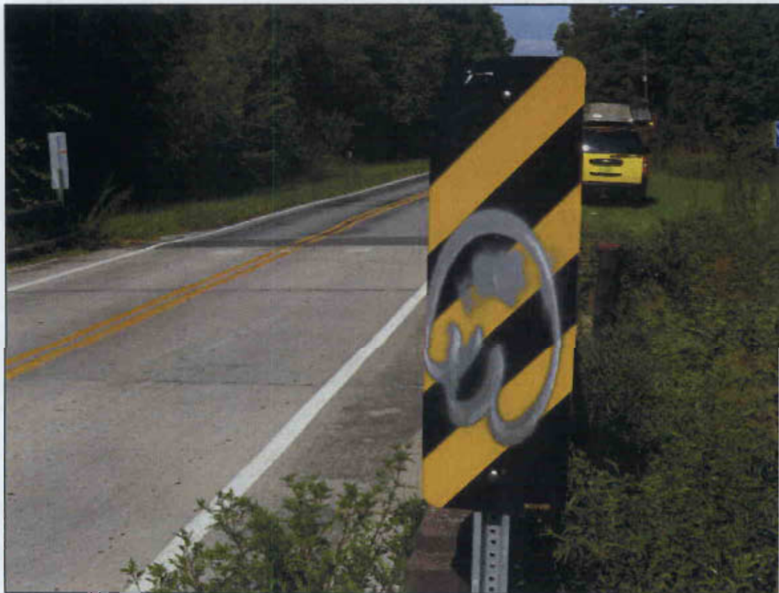
NORTHEAST DELINEATOR DAMAGED
